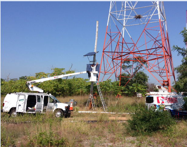
Setting up Solar Panels at Pleasure Beach.
